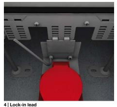
4) Lock-in lead Device carrier with CEE socket and box in lock-in lead suitable for floor constructions from 160 mm. Always use the lowest locking position. Clamp device carrier firmly with a socket head wrench.
