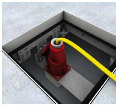
**6 | Straight connector** When using a straight connector, note that the cover cannot be closed while in use. Protect installation unit – accident risk!
